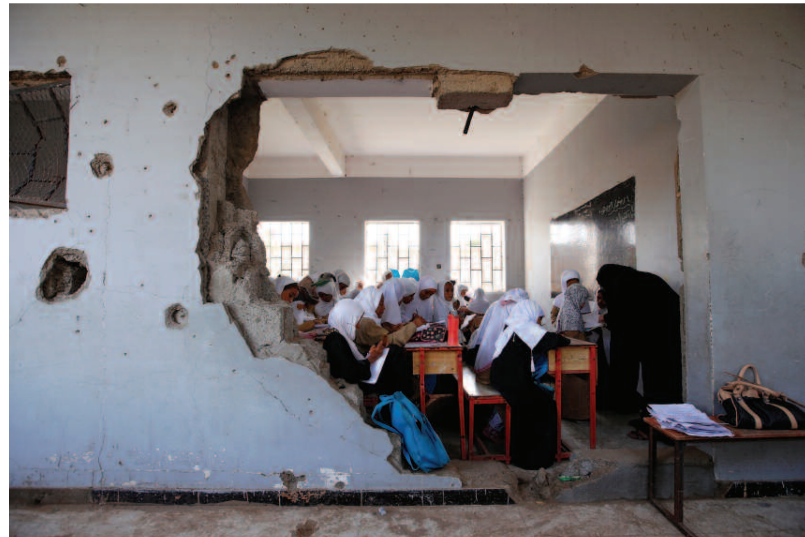
Girls attend school in the Red Sea port city of Hudaydah, Yemen, on October 24, 2017. The school had recently been damaged by an air strike.
